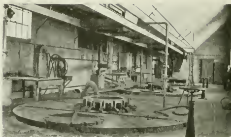
Fig. 15.—Charging Floor of Digester House.
